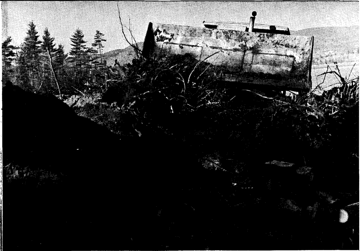
Bulldozer must clear obstruction along the shore of Squam Lake before fill can be trucked in and smoothed. Trees and large boulders pose the biggest problem to the establishment of the "1/2 mile of beach." (photograph by Malcolm Taylor)
